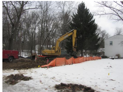
New House Construction on Revere Road former razed lot
